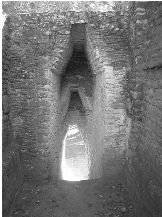
Figure 3. Mayan corbel arch from Cahal Pech, Belize, 900 BC (picture by Clark Anderson/Aquaimages under the Creative Commons License [3]).
